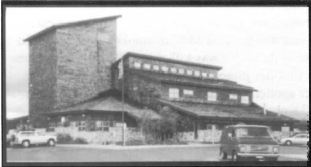
View of the McCall Smokejumper Base Headquarters. It is an outstanding facility.
