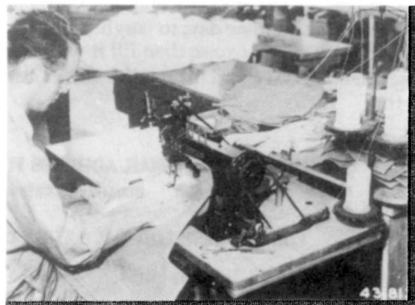
A Singer Model 121, four-needle sewing machine, at the Missoula Base, 1945. Photo courtesy of the U.S. Forest Service.
